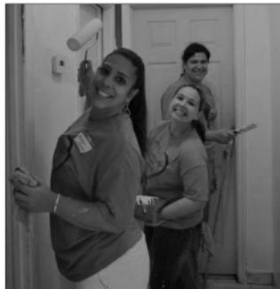
A home in Florida City is painted, inside and out!
