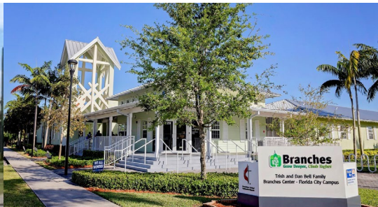
The Trish and Dan Bell Family Branches Center - Florida City Campus which opened in the Fall of 2014
